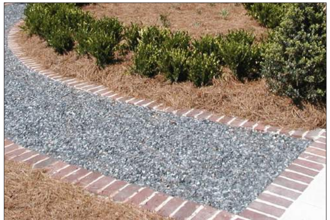
Crushed shale with brick edge
