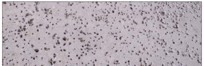
Rock salt finished concrete
