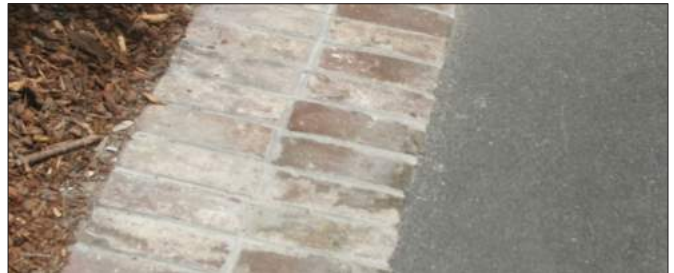
Brick edging on asphalt driveway
