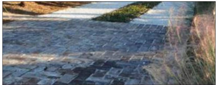
Brick driveway apron and crushed stone carriage tracks
