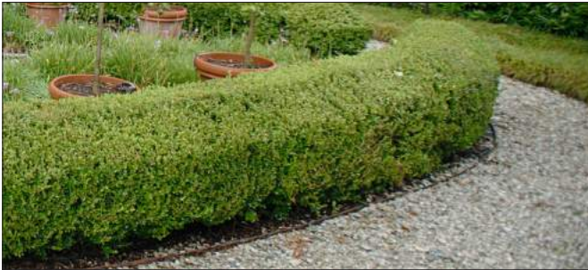
Metal edging used to retain loose stone on a path
