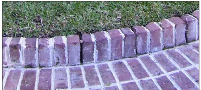
Brick edging on a brick walkway
