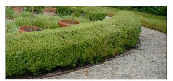
Metal edging used to retain loose stone on a path
