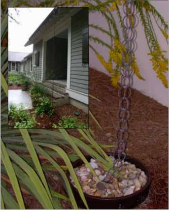
Detail: Rain chain in splash area of loose stone
