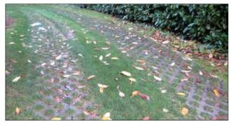
Carriage tracks with pervious pavers
