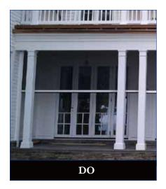
Install retractable screen enclosure tracks on the inside face of the columns.
