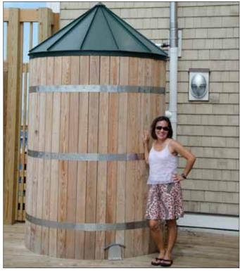
Example of a 10' tall above ground wood sided rain barrel
