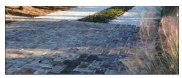
Brick driveway apron and crushed stone carriage tracks
