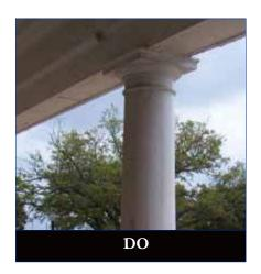
Column and beam support the roof.
