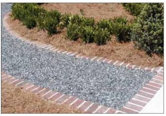
Crushed shale with brick edge
