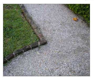
Loose sand, shell, and stone held in place with brick edging
