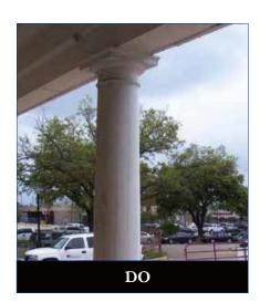
Shaft nearest top of column aligns with face of beam.
