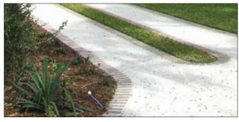
Carriage track drive with brick edge and seeded aggregate
